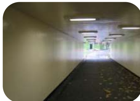
Concrete surfaces of a subway were mechanically abraded, primed with 503 SPEP and top coated with 508 UVPU
