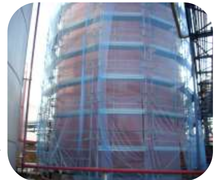
Petrol storage tank at European refinery hydroblasted and coated with 2 x coats of Resichem 555 Resinox
