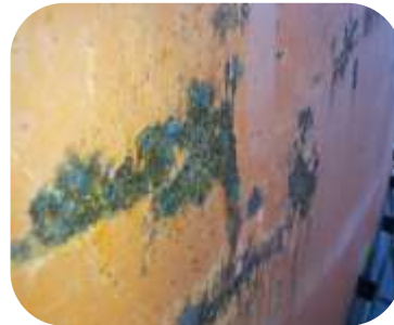
Petrol storage tank at European refinery hydroblasted and coated with 2 x coats of Resichem 555 Resinox
