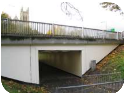
Concrete surfaces of a subway were mechanically abraded, primed with 503 SPEP and top coated with 508 UVPU
