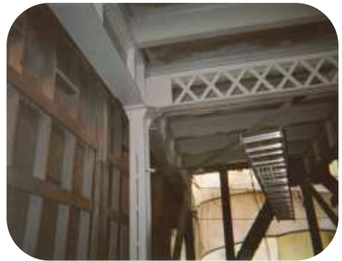
Structural steel underneath a water tank abrasive blast cleaned and coated with Resichem 501 CRSG
